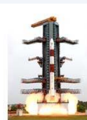
Second Launch Pad Count Down Checkout System
