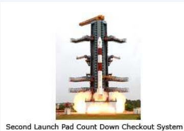
Second Launch Pad Count Down Checkout System
